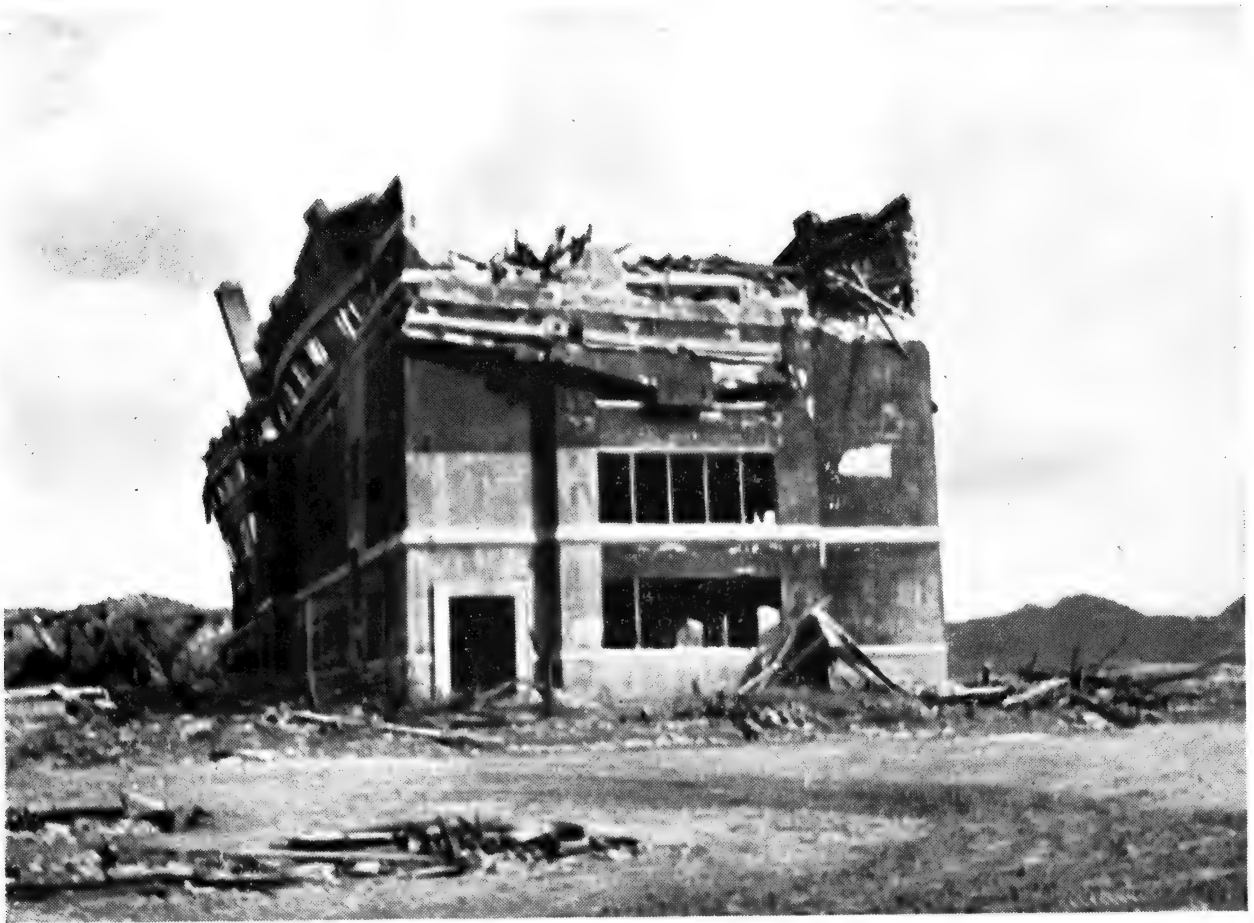
Photo No. 5. NAGASAKI. Reinforced concrete school with a timber roof, 500 yds. from the centre of damage, which is to the right of the photograph. The upper part of the long wall further from the explosion has been bent over, partly by a thrust through the roof from the other long wall and partly by wind suction. This is a typical case of "mass distortion." See paragraphs 15 and 22.
